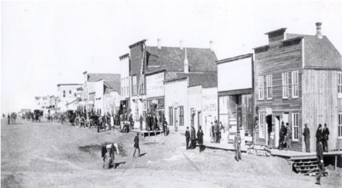
Enid under construction November 1893. the Streets had not yet been leveled
